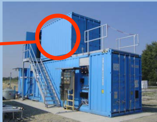
LMBV Schwarze Pumpe Germany, 5 MPPE units, 75 m3/h; Ar, Al, PAHs
